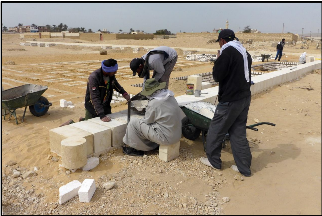
Figure 1: A group of the builders laying a corner block at the south-east corner of the Long Temple. View to the north. Builder Shahata Fahmy is seated with his back to the camera.
