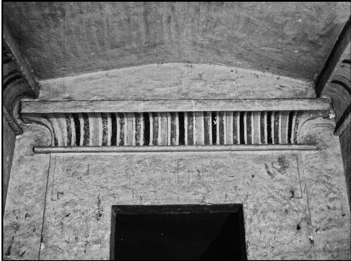
Figure 14: The doorway to Any's shrine, showing the remains of the texts and figures of Any put in place by an outline draftsman. Photo by Gwil Owen.
