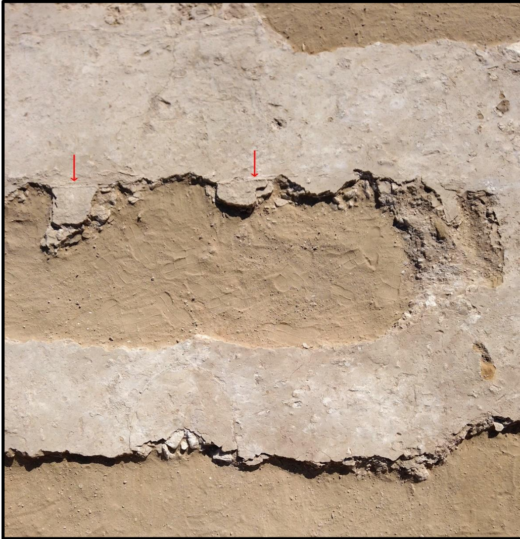
Figure 22: The picture shows the surface of the gypsum-concrete foundation layer at the entrance system before the western large offering-table. It illustrates how the ancient demolition process worked. The talatat -blocks have been removed along the length of the wall (the red arrows point to impressions in the original mortar from the edges of the wall). The next stage was to cut away the foundation concrete from where the wall had been. This had been done by cutting narrow parallel trenches from side to side. A pair of unfinished trenches is at the right edge of the picture. North is towards the left.
