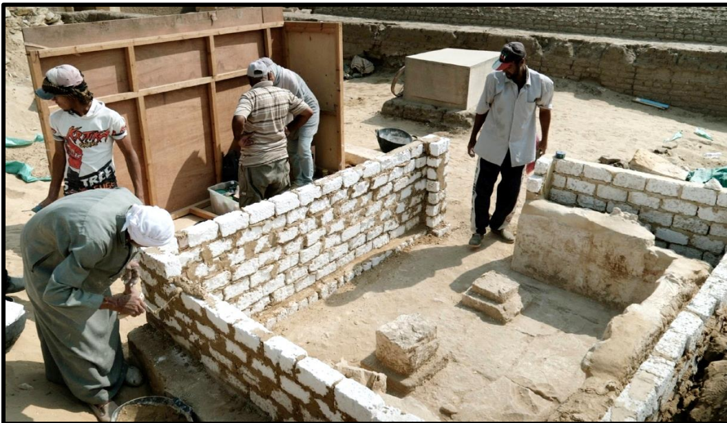
Figure 9: Constructing the protection for the Little Chapel (photo: Servass Neijens).
