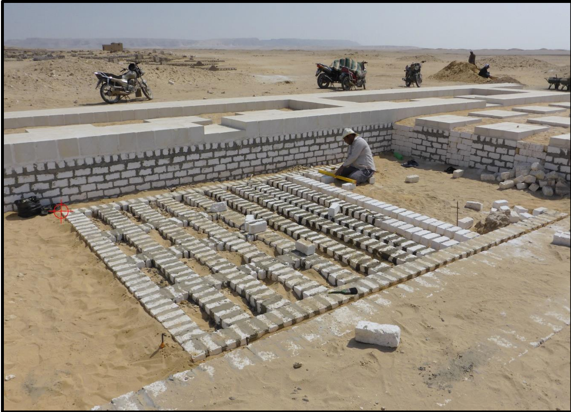
Figure 15: The site of the eastern large offering-table and the lowest course of new stones being laid. Beneath the target symbol in the top left (north-east) corner of the new foundations lies a patch of the ancient foundations where traces of gypsum mortar mark the original corner of the offering-table. View to the south-east.
